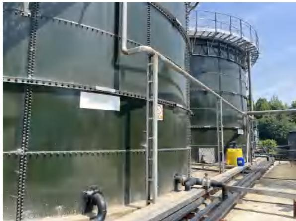
二级硝化/反硝化罐+一级硝化罐（接地罐体）
